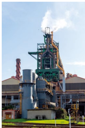
Clean Safety Valve(yellow) installed in Gwangyang Steelworks furnace#1
